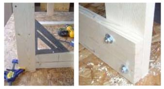
two  $\frac{1}{4}$ " holes for carriage bolts. Holes should be drilled in a diagonal. Insert the carriage bolts from the outside, and attach a washer and nut on each.
