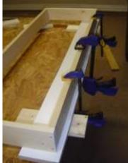
connect these two pieces together. Be sure that the screws are not longer than about  $\frac{3}{4}$ " so they do not go all the way through the desk top or the 1" x 4". It is recommended that the screw holes in the desk top be predrilled. See picture above.
